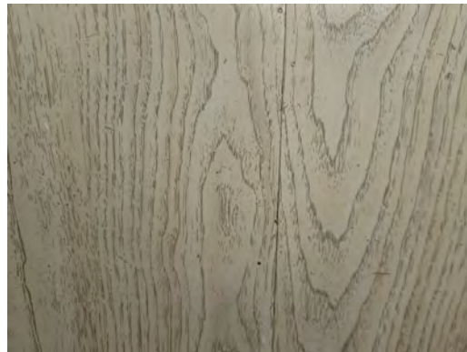
884-12 Laminate Wall Paneling Interior 2 nd Floor
