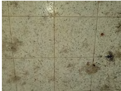
884-10 Rolled Flooring/Mastic Interior 2 nd FI Bathroom
