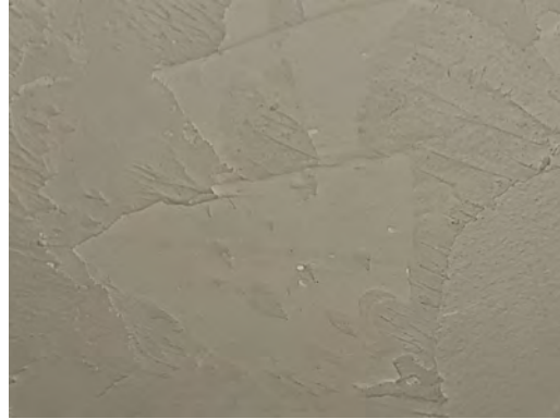
884-8 Drywall/Joint Compound Typical Interior Walls/Ceilings
