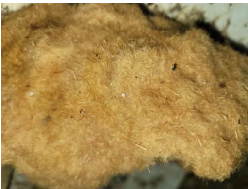
884-5 Insulation Typical Interior
