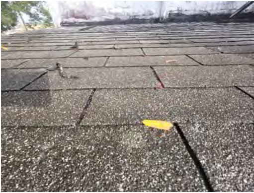
884-1 Asphalt Shingle Typical Exterior Roof
